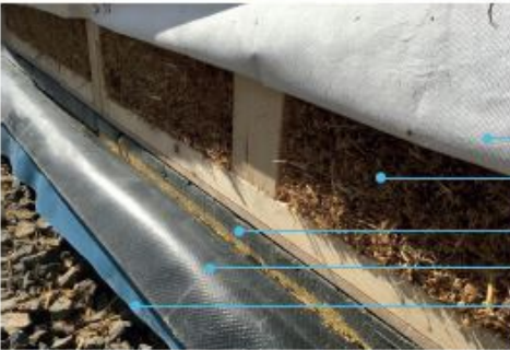
Figure 8.23 Perimeter sole plate fixed to the concrete slab and EPS filler on top of the edge insulation piece (top).
