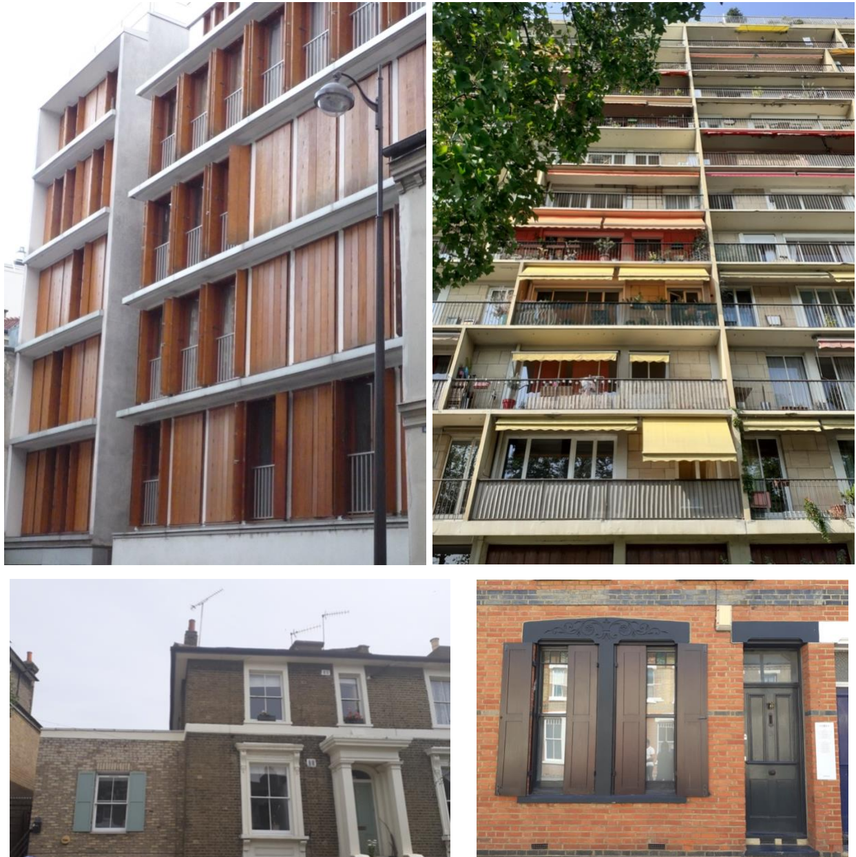
Figure 34: Examples of movable shading devices. They are used differently across the facade, showing user adaptation and individual preferences; these features can reasonably easily be part of a retrofit. On the bottom left image, external shutters were included in the side extension to the original Georgian house, in a Conservation area.
