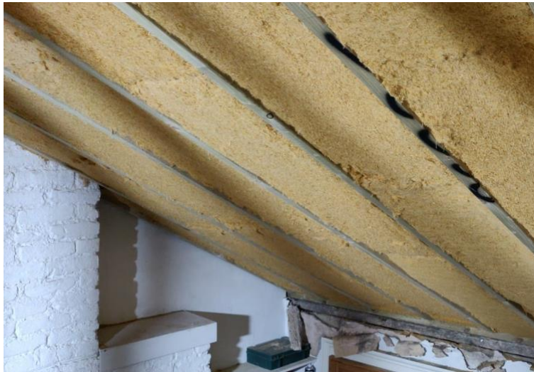
Figure 43: Wood fibre roof insulation being applied
