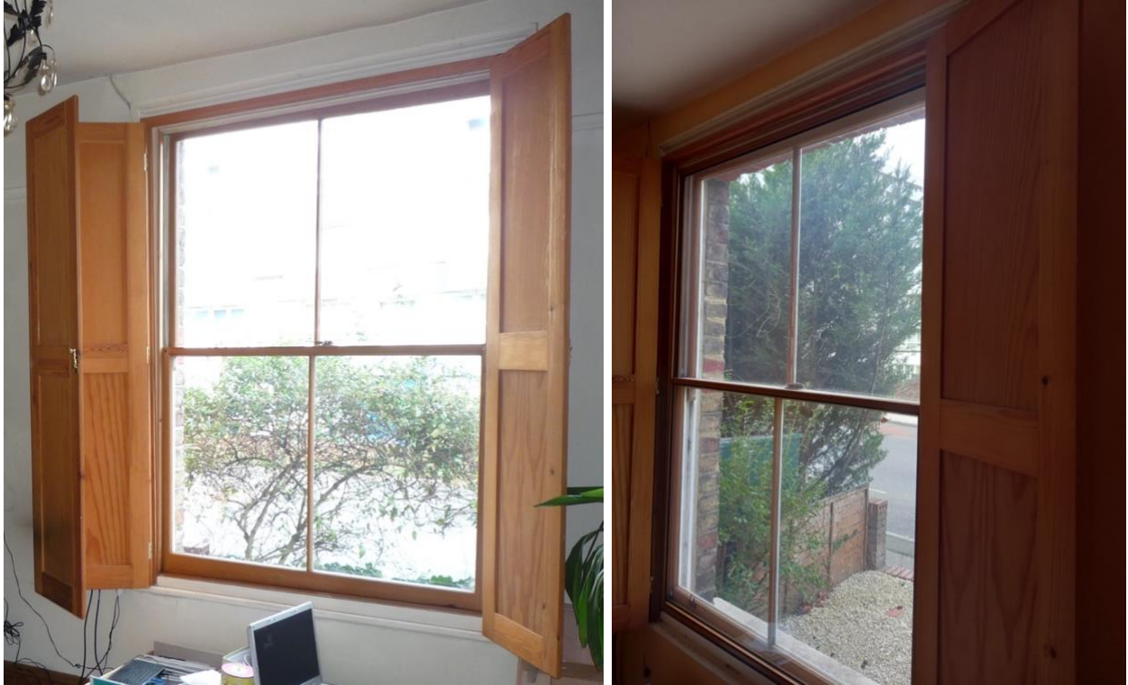
Figure 40: Example of secondary glazing added to sash window: (left) before, (right) after: the bespoke secondary glazing was made to match the lines of the original, and the bottom pane slides up, but the overall opening is likely to be less effective compared to the highly effective bottom & top openings possible from original sash windows. Thanks to the slimline profile of the secondary glazing, it was possible to retain the internal shutters.
