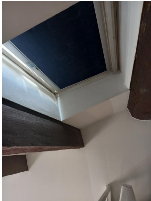
Figure 37: Openings may be available on paper, but in practice difficult to access or operate due to their design, or because the system or feature to operate them is lost or broken e.g. left: a long stick is missing to reach the handle of the high-level opening; right: opening the velux window in this loft conversion involves climbing on the bed and precariously bending over the mezzanine balustrade.
