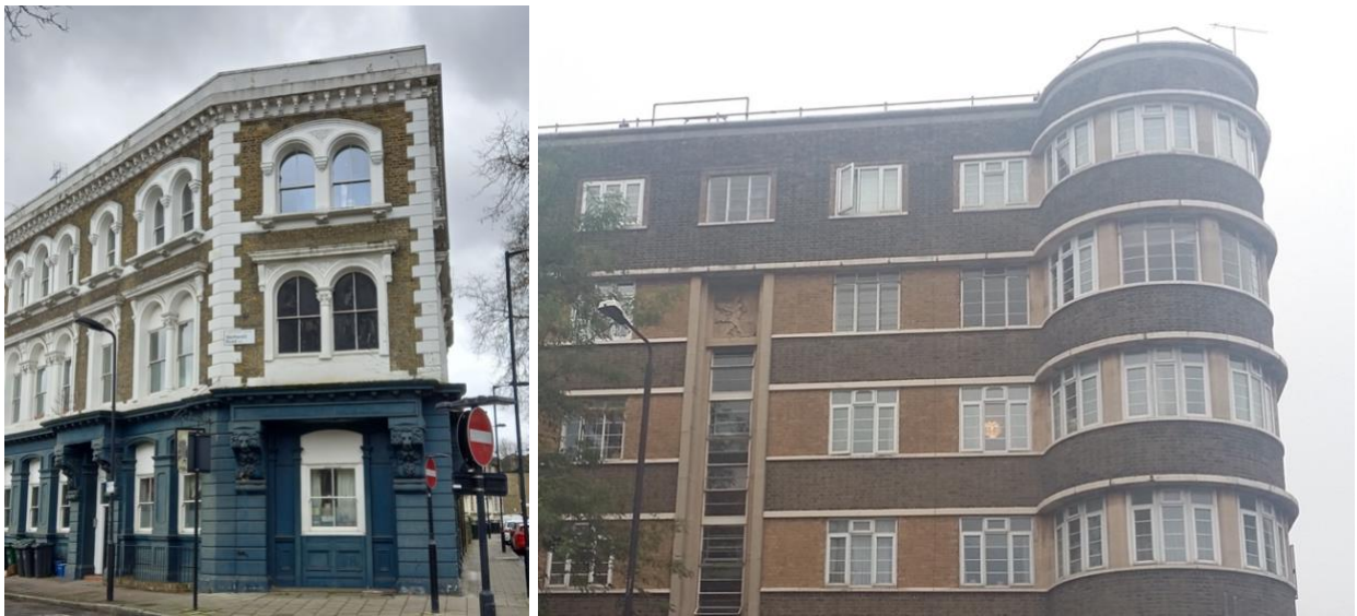
Figure 29: Example of glazing proportion between 35% and 50% of façade area. These also illustrate situations where it is useful to check the glazing proportion in relation to floor area, not just façade, as reasonable proportions in relation to façade length could still result in high proportions in relation to floor area: corner dwellings, high ceilings, and highly articulated facades with features such as bay windows
