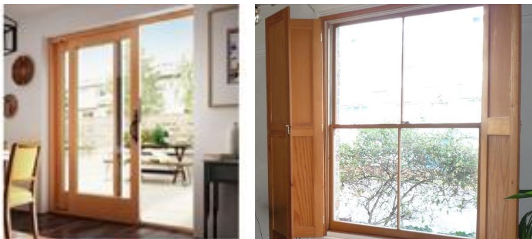
Figure 38: Examples of openings providing just under 50% free area: sliding patio door, sash window.
