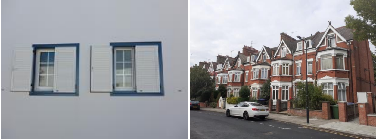
Figure 16: On the left, example of light-coloured (high albedo) facade, likely to be of lower temperatures than surfaces such as brick, as in the example on the right where dark brick south-facing walls could reach high temperatures.
