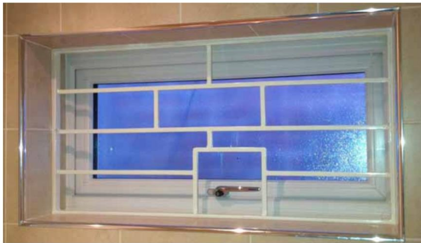
Figure 13: Examples of secure window openings. These measures could easily form part of a retrofit project, if not already installed on the existing windows.
