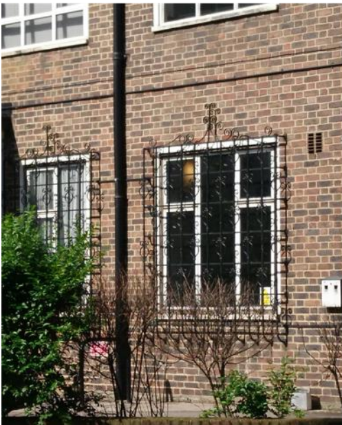
Figure 13 (continued) Examples of secure window openings. These measures could easily form part of a retrofit project, if not already installed on the existing windows.
