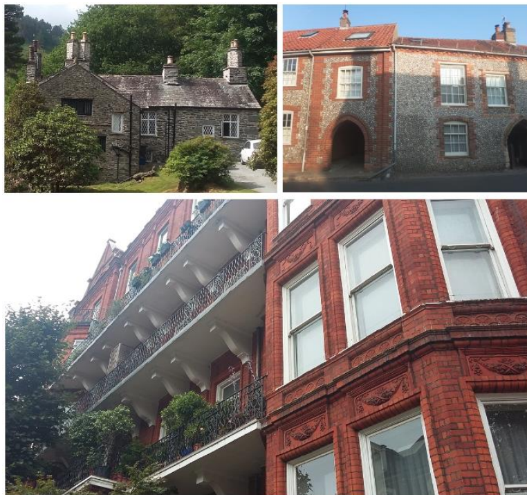
Figure 24: Buildings of traditional construction often have exposed thermal mass, for example with walls made of stone or solid brick, with the mass left exposed or covered by materials such as lime or clay plaster which retain its benefits; the mass may however have been covered by subsequent internal works using plasterboard or other light-weight materials, so this should be checked before scoring the mitigation points in this question.
