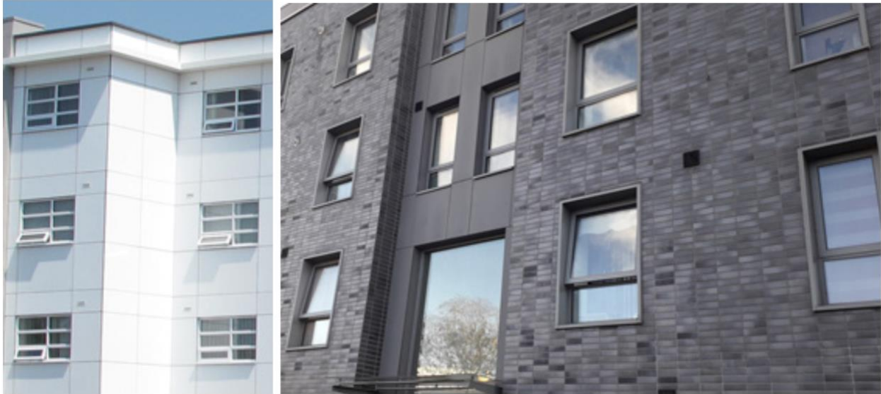
Figure 36: Examples of restricted window openings - left): Only one of six panes was openable, and only to a limited extent - the flats overheated (GHA Preventing overheating report, 2014); right: only the top 2/3 part of windows opens, and the opening is restricted to only a very small gap.
