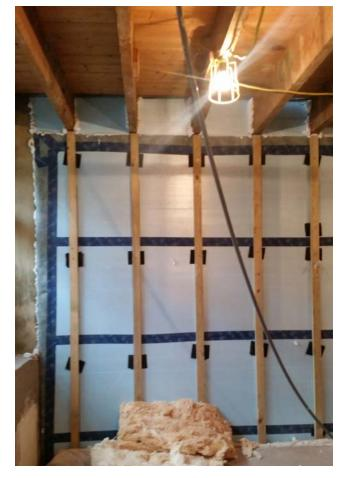
Figure 6.35 - Internal wall insulation to original external building envelope which was mostly cavity but solid in isolated location, Marion Baeli and Robert Prewett
