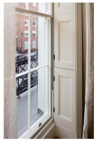
Figure 6.29 - High performance secondary glazing post retrofit. Prewett Bizley Architects
