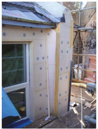
Figure 6.12 - Installation of external wall insulation - BBM Sustainable  $\ensuremath{\mathsf{Design}}$
