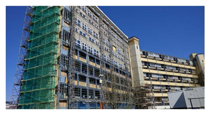
Figure 6.14 - Courtyard side during construction, showing new EWI and triple-glazed windows being fitted. ECD Architects.
