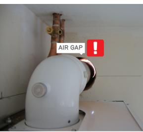
HEAT LOSS THROUGH UNINSULATED PIPES
