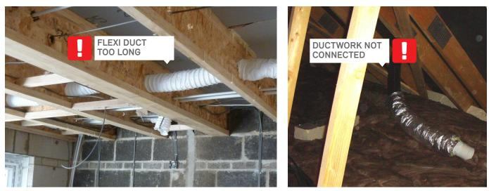
FLEXI DUCT TOO LONG AND NOT SUPPORTED = FANS WILL BE NOISY / INEFFICIENT VENTILATION COMMISSIONING NOT DONE CORRECTLY
